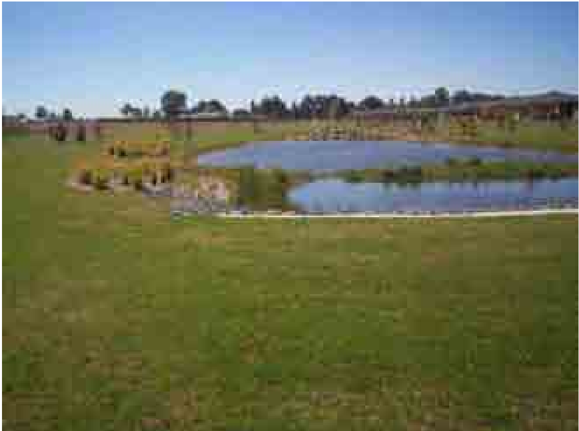
Neil Algar Reserve and the stormwater retention pond in the southern half of the reserve
