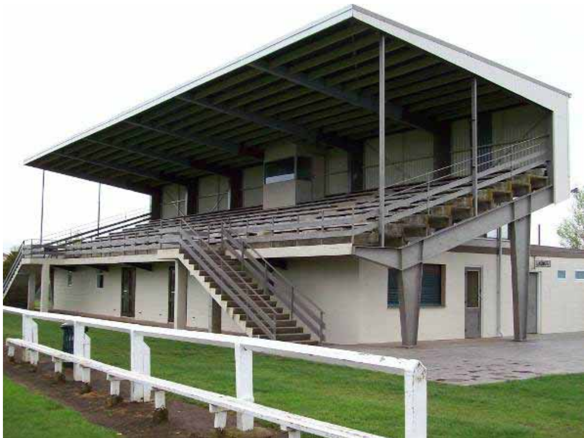
The A.R. Johns Memorial Grandstand
