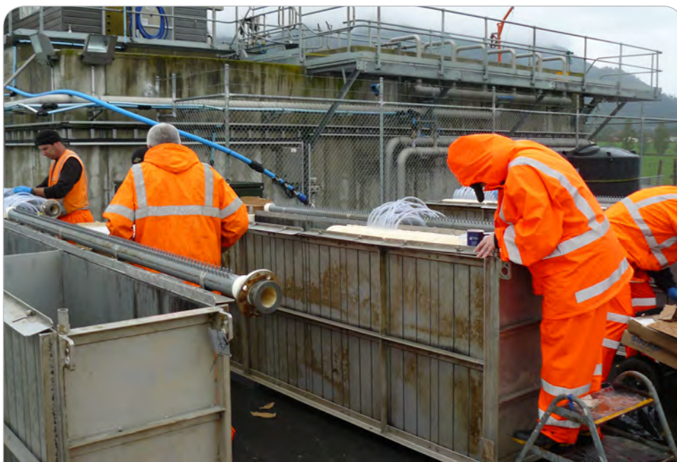
Staff replacing the membranes at the Te Aroha Wastewater Treatment Plant.
