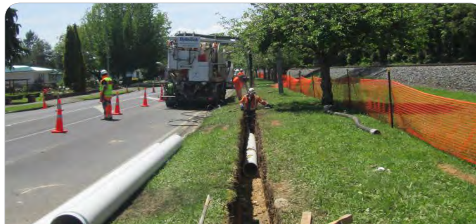
Stormwater pipe renewals on Firth Street, Matamata.
