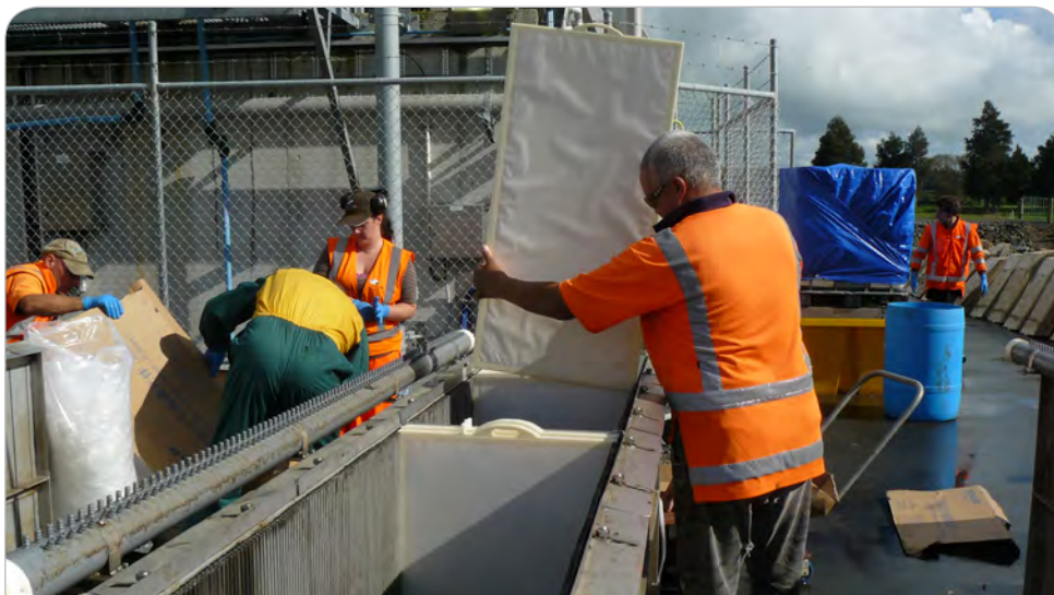
Membranes being replaced at the Te Aroha Wastewater Treatment Plant.
