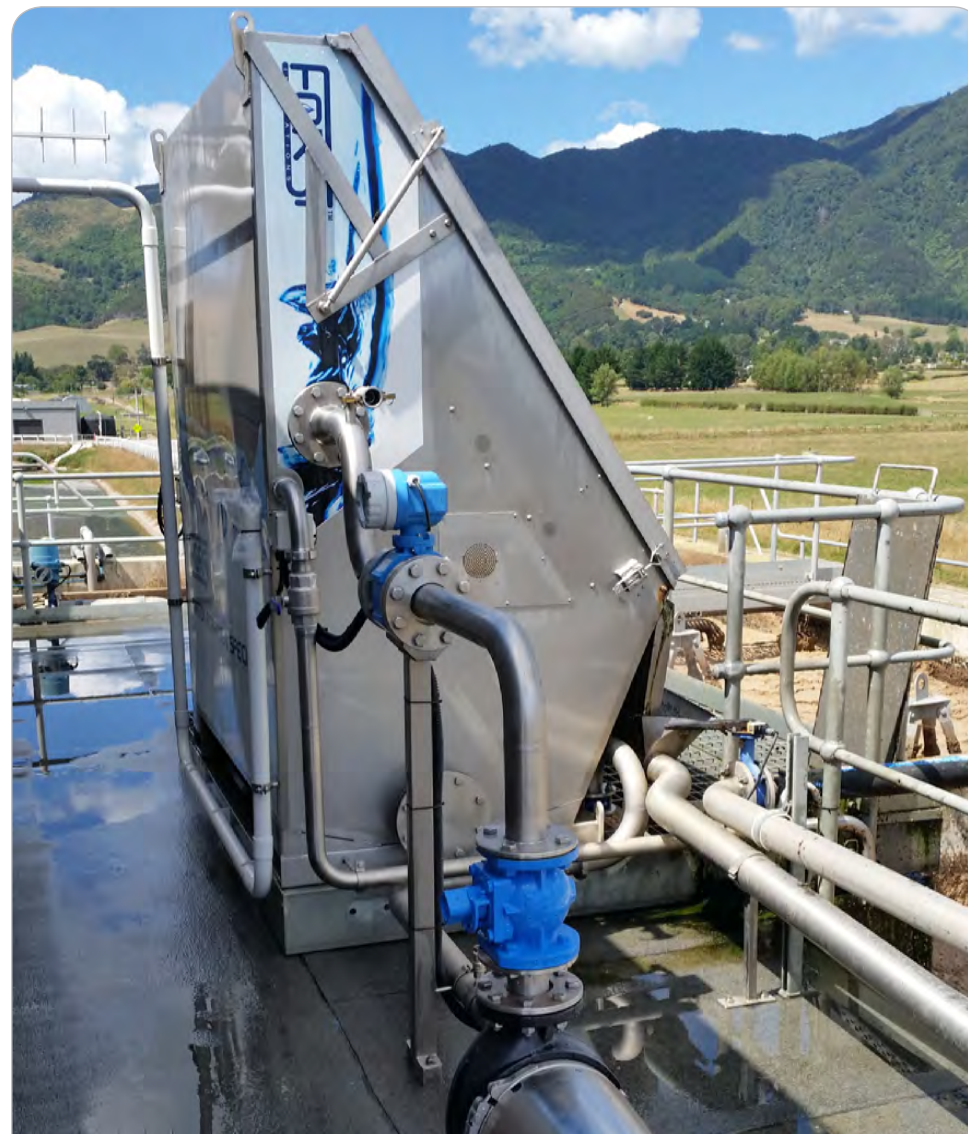
Rotary screens, Te Aroha Wastewater Treatment Plant.
