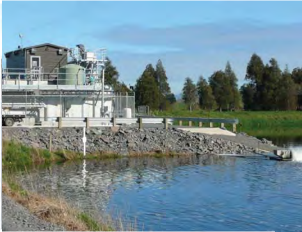
Wastewater treatment plant – Te Aroha
