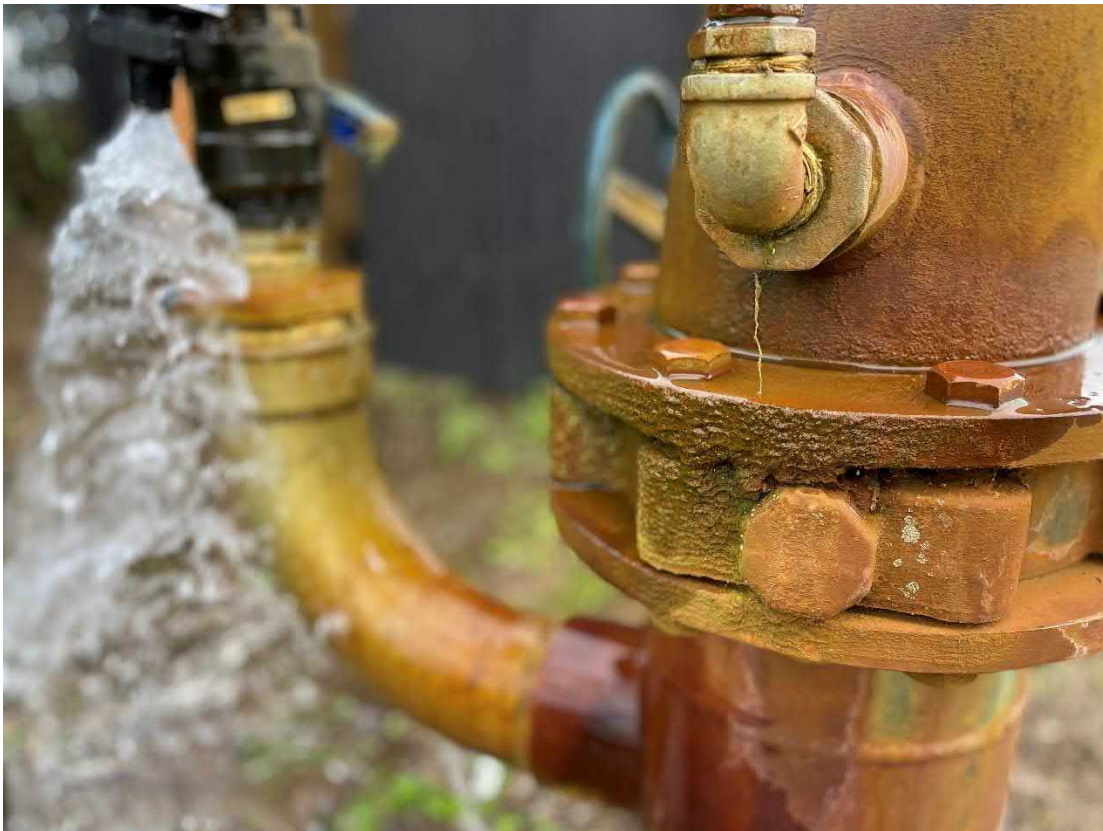
Figure 3: Sampling Point on Java Bore (72_6680) Showing Iron Staining.
