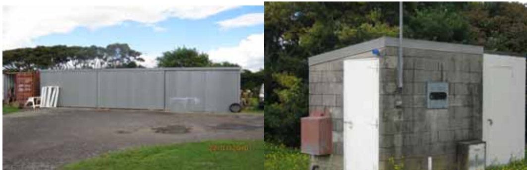
Photos 9 and 10 Implement Shed and Pump Shed
