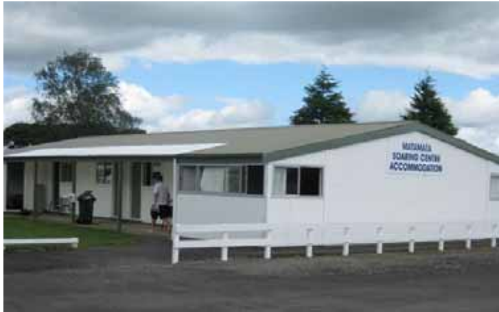
Photo 6 Matamata Soaring Centre Accommodation Block
