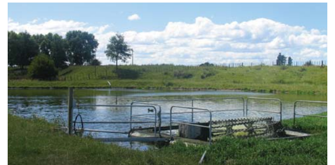
The current Wastewater Treatment Plant at Waihou
