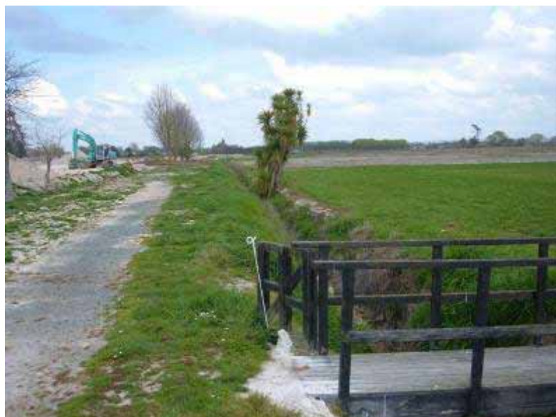
Figure 49: A footbridge over a boundary drain.
