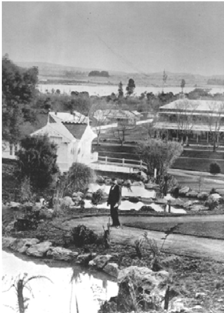
Lakelets behind the Cadman Building from Te Aroha Domain Conservation Plan c/o Matthews and Matthews Architects Ltd.
