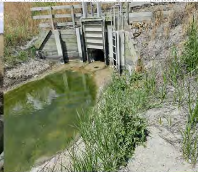
▶ PIAKO PUMP STATION
